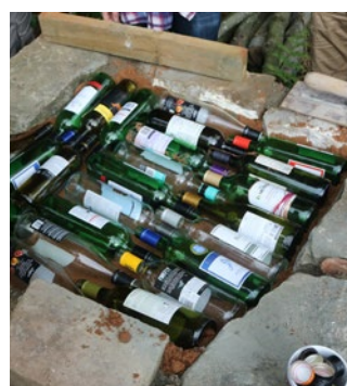
First, construct a sturdy plinth, then ensure that the top surface is flat, fireproof and heat resistant. Old bottles bedded in sand help to insulate the plinth and are topped with more sand and old bricks from a storage heater.
